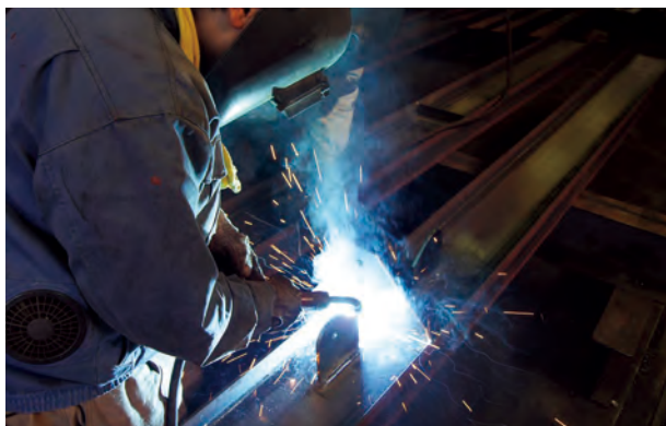
Welding operation at the factory
