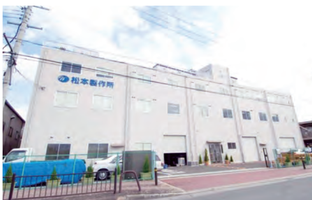
Exterior of the headquarters
