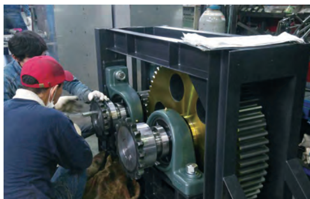
Frame production install operation
