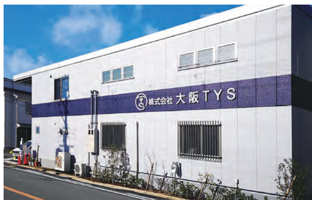
Exterior of headquarter
