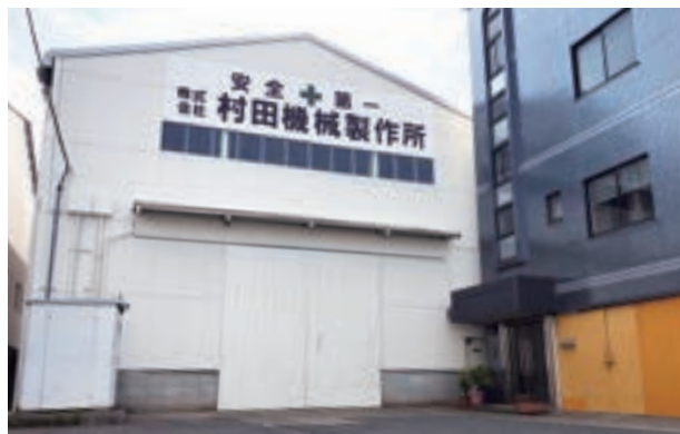
Head office and factory at Yao city in Osaka
