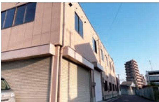
Headquarters plant for integrated handling of prototypes, etc.
